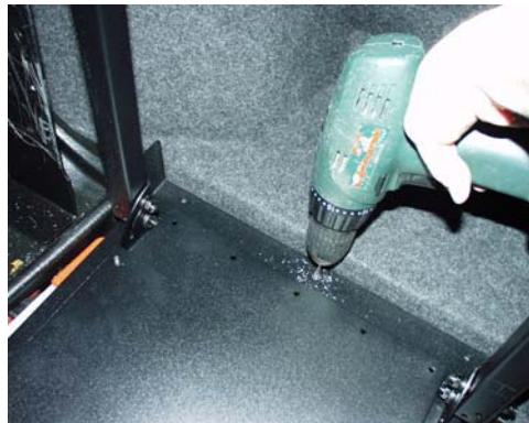
Pre-drill lower mounting holes using 1/8" drill bit and attach with #10 x 3/4" Sheet metal screws
